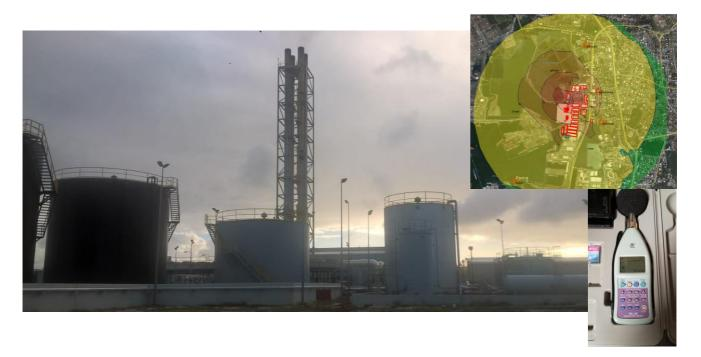
Rationale: Aqualectra has asked EcoVision to perform noise measurements and modelling of sound immissions at their Dokweg II-A diesel power plant. Aqualectra required a noise investigation in order to comply with their environmental permit.
